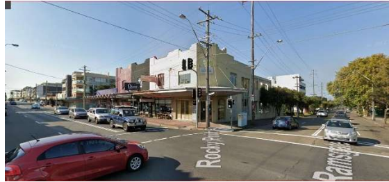
Figure 33 - North eastern corner of the intersection, including early shop top housing.
