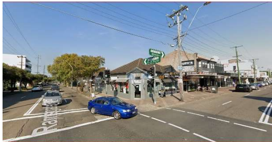
Figure 34 - A single storey corner property on the south eastern corner.
